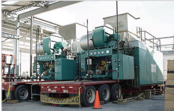
While a new steam plant was being constructed, process steam and the steam provided to the neighboring plant could not be interrupted. To ensure this, two complete and independent 70,000 lb/hr trailer-mounted boilers were supplied for temporary use, providing 100% redundancy.
