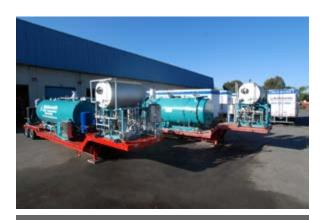
TRAILER MOUNTED BOILERS Figure 2. The typical configuration of an open-trailer mobile steam plant consists of a water tube mounted to a trailer for mobility.
