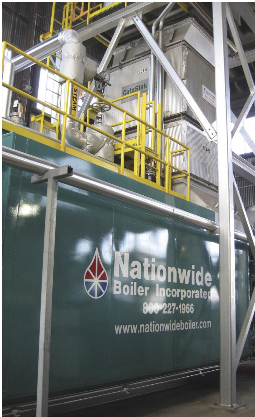
A reconditioned 70,000 lb/hr boiler with SCR was sold to a customer in California and installed on-site.
