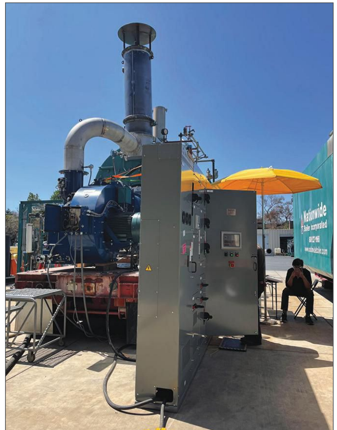
Figure 1. Testing of a new PLC-based motor control panel with remote monitoring capabilities.
