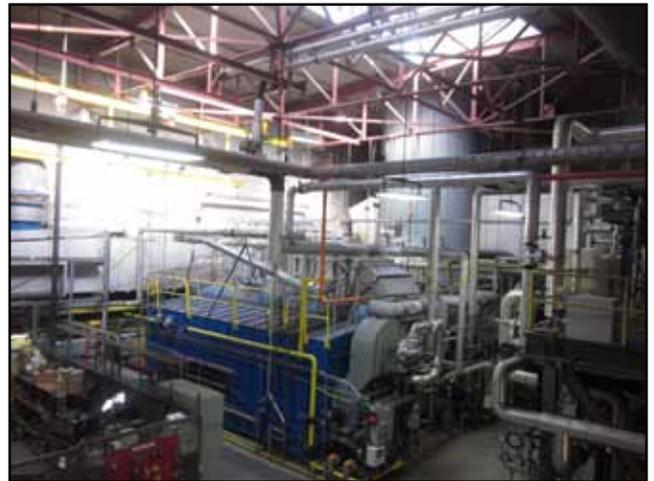
Two (2) 55,000 lb/hr watertube boilers with a single Ammonia-Free CataStak™ SCR system.
