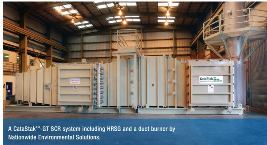
A CataStak™-GT SCR system including HRSG and a duct burner by Nationwide Environmental Solutions.
