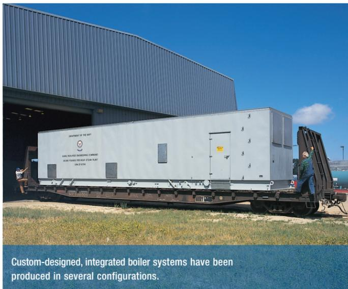
Custom-designed, integrated boiler systems have been produced in several configurations.
