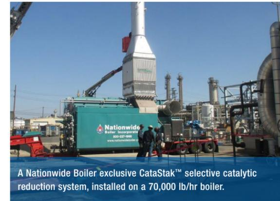
provides flexibility with the option of utilizing anhydrous ammonia, aqueous ammonia, or a 32.5% liquid-urea solution (otherwise known as DEF).
