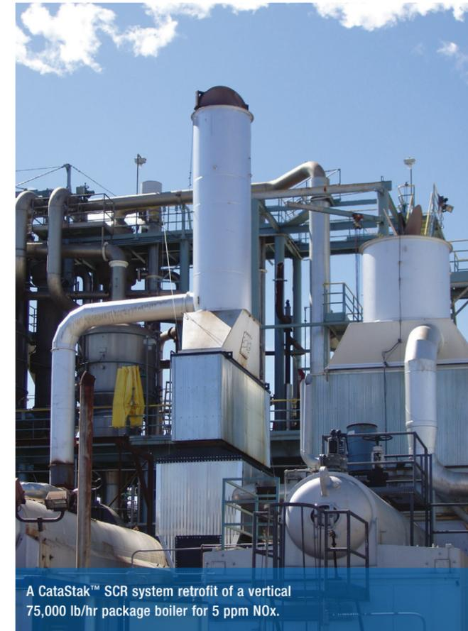
A CataStak™ SCR system retrofit of a vertical 75,000 lb/hr package boiler for 5 ppm NO<sub>x</sub>.
