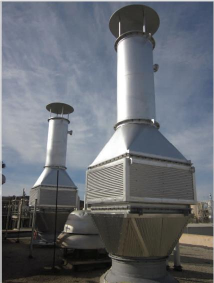
Overall, the advanced Ammonia-Free CataStak™ SCR system easily reduced NOx emissions from 30 ppm to less than 3 ppm NOx with ammonia slip under 2 ppm. The system also complies with Rule 1146 without concerns about meeting future NOx emission limits, providing PDC with superior NOx performance and hassle-free, dependable operations.
