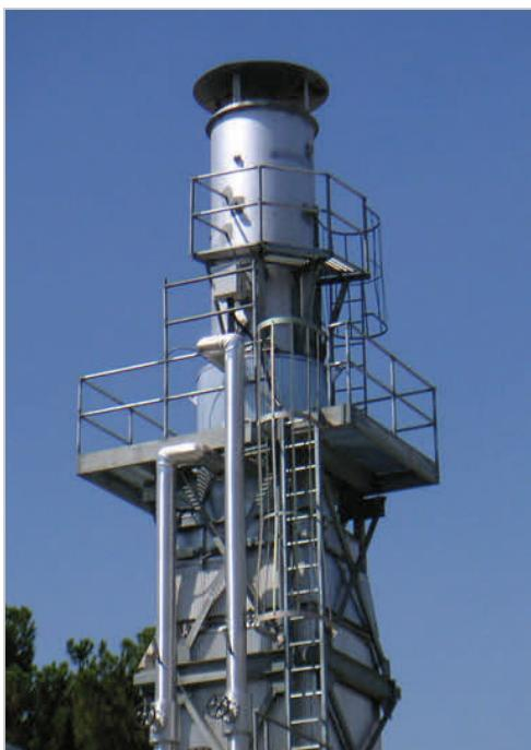
The equipment easily met the 5 ppm ultra low NOx emission requirements, which ensures that the customer will meet future NOx emission limits required by the local AQMD. The newly installed EconoStak economizer reduced stack temperature from 450°F to 300°F, resulting in a nearly 4% increase to the current boiler's overall efficiency and an immediate energy cost savings.
