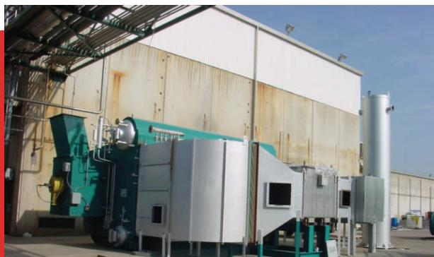
A 50,000 lb/hr boiler supplied with a low NOx 30 ppm burner, CataStak™ SCR system and EconoStak economizer. The unit was certified to operate at better than 95% fuel-to-steam efficiency.
