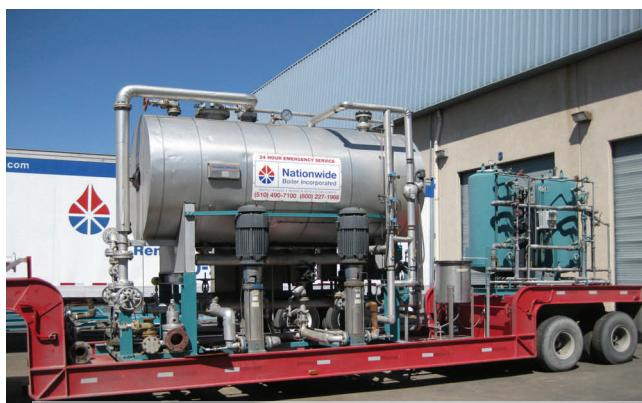
A 30,000 lb/hr mobile feedwater system includes a deaerator, pumps, controls and water softener.
