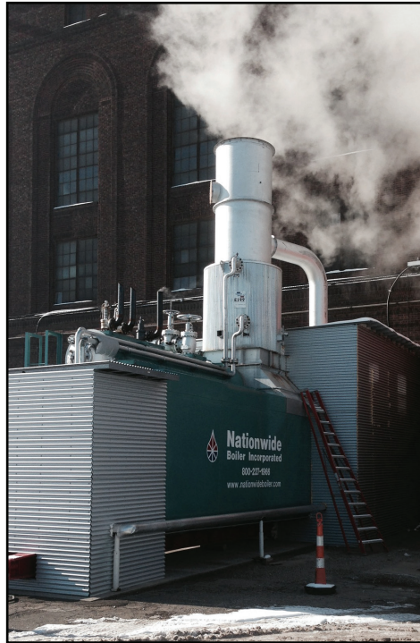
82,500 lb/hr Trailer-Mounted Rental Boiler and EconoStak Economizer Surviving the Cold
